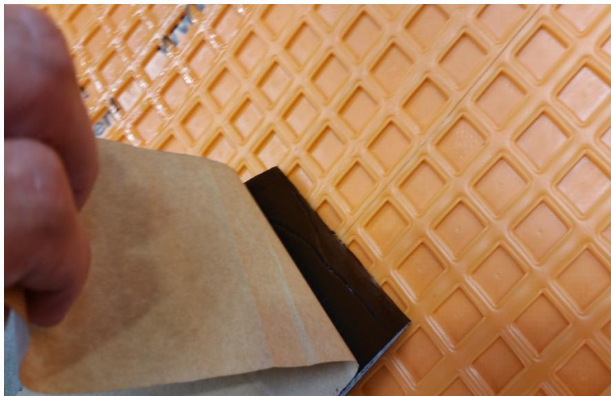
Install the Ditra Flash 80mm Tape covering all sheet joints, using a roller compressing the tape into the sheet removing backing paper down the length of the joint.
