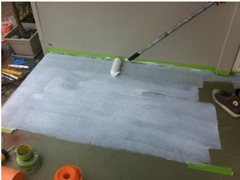
Apply PSA (Pressure Sensitive Adhesive) to the substrate or approved membrane with a 8 nap Roller. Allow PSA to tack off (changes colour from milky to clear). PSA once tacked off, becomes permanently tacky, allowing the schluterDITRA to be re-aligned upon laying – or lifted to inspect the waterproofing membrane multiple times without having to reapply adhesive.
