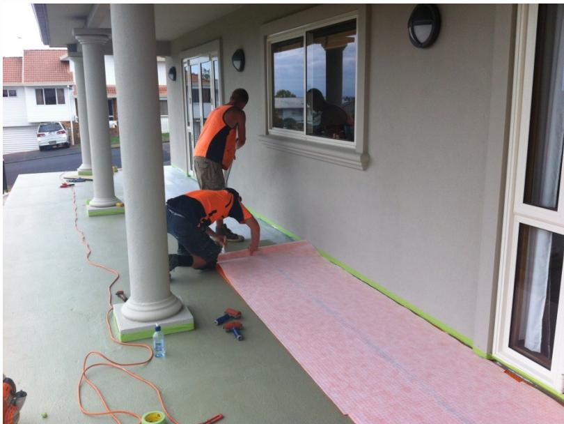
Lift up a corner of the matting to check coverage. Proper installation results in full contact between the fleece webbing and PSA adhesive.
