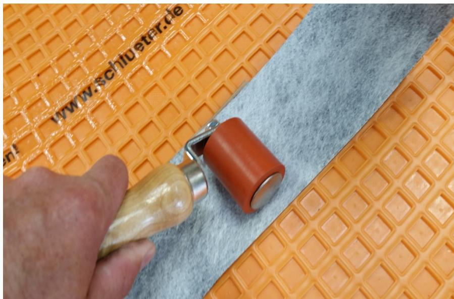
Tile can be laid on the installed schluterDITRA immediately using Laticrete 4XLT Tile Adhesive, and Laticrete Epoxy Grout. The installation of tile must be laid back buttered also insuring full coverage of adhesive, fulling dove tail cavities of the Ditra troweled flush with the reverse side of a notched trowel.
