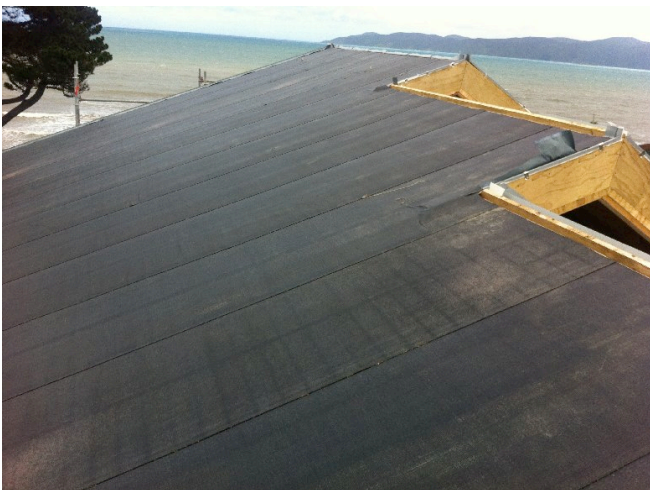
BituBOND installed under tiles
