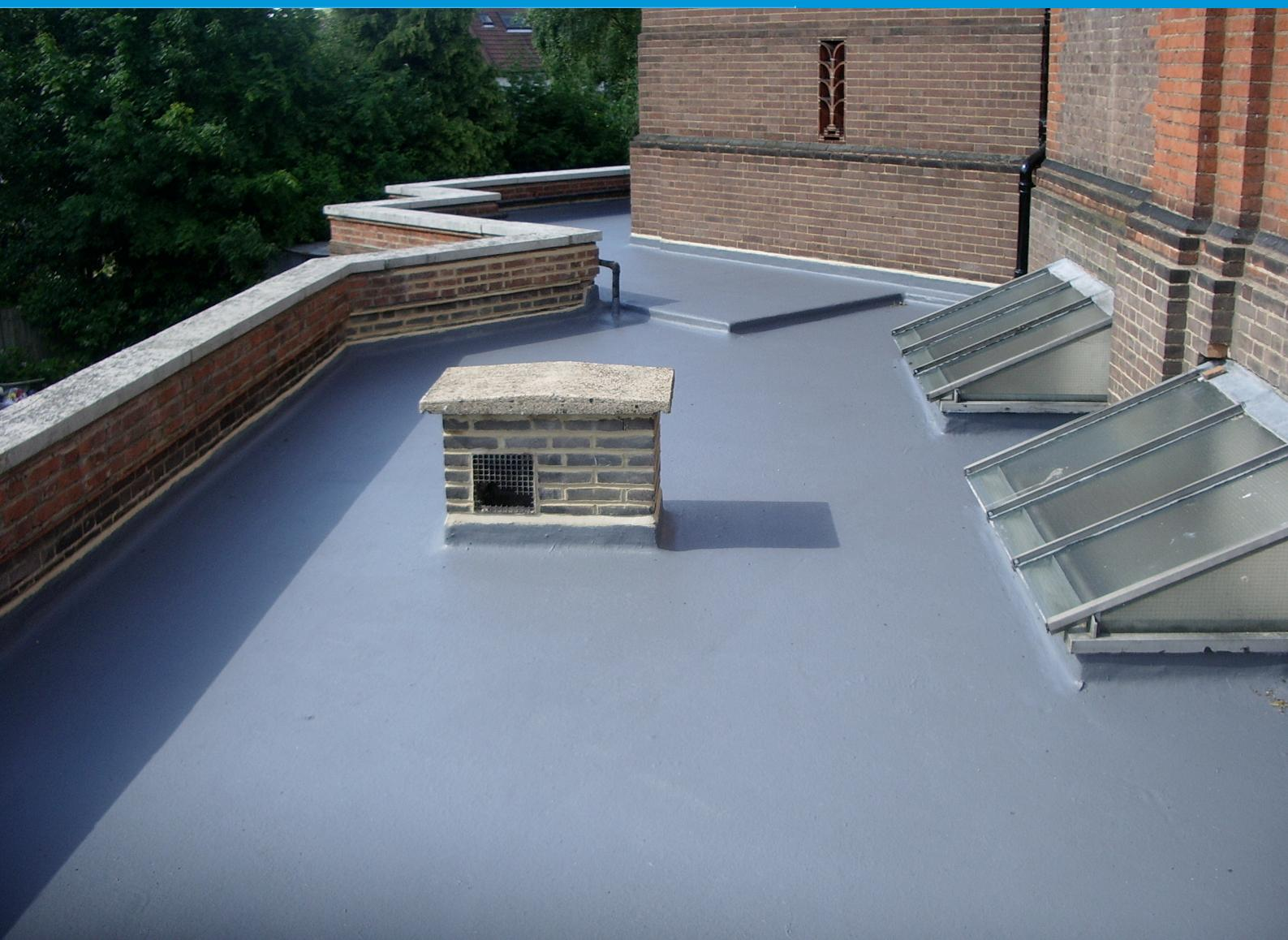
Polyurethane Re-Roofing Liquid Membrane
