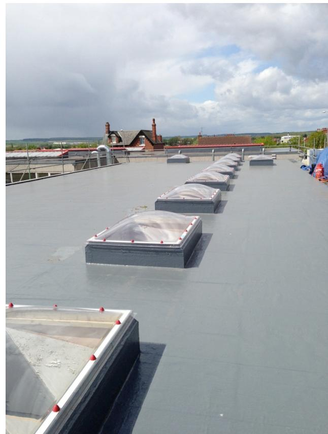
PolySEAL is an ideal solution for re-roofing and remedial repairs on existing membrane roofs. Old membrane roofs can be easily re-coated and brought back to a new standard with minimal disturbance to the existing roof or structure.
