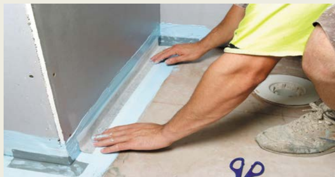
Above: Elastoproof detailing with Gripset 38®
