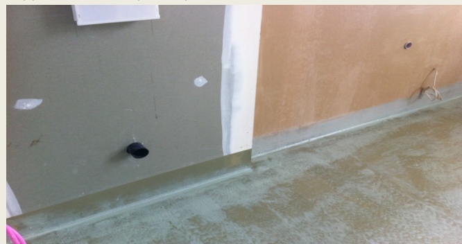
Gripset 2P® Internal Waterproofing
